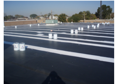
Lucas #6000 is ideal for EPDM seam restoration. Can go over cover tape. Available in black for seams only or white for full roof restoration as shown.
