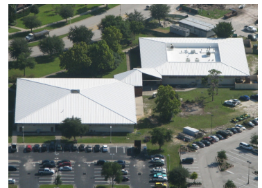
Energy Star White on metal and asphalt BUR. One solution for multiple roof surfaces.
